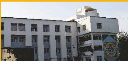
ST. KABIR SCHOOL DRIVE-IN (A)
